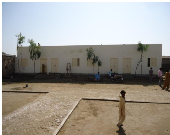
View of New school building at Bahadur
